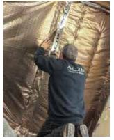
All finished edges should be stapled every 50mm and secured with tape and batten.
