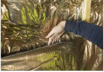
2 Fix adjacent layer overlapping by 50-100mm. Staple to timber support, and seal joint with **ACTIS tape**. Cut **HCONTROL HYBRID** oversized at floor and ceiling, allowing it to be adequately sealed by a batten. All finished edges should be stapled every 50mm and secured with tape and batten.
