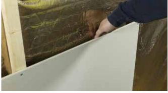
Around windows and doors, seal **HCONTROL HYBRID** with **ACTIS tape** and batten. Seal around any cable or pipe penetrations with **ACTIS tape**.
