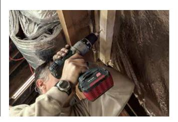
Prepare for plasterboard by fixing horizontal or vertical battens (ACTIS recommends 38 x 38mm to gain full thermal performance) nailing through **HCONTROL HYBRID** to the rafter.
