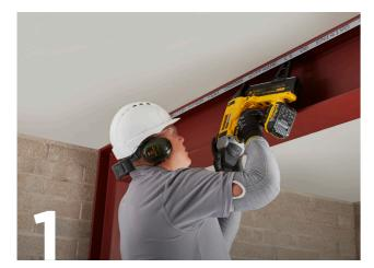
For two or three-sided protection to steel beams or columns, secure Gypframe FEA1 Steel Angles to both sides of the wall / soffit flange using appropriate fixings.
