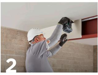
Cut Glasroc F FireCase boards to width and use Glasroc F FireCase Screws to fix to the Gypframe FEA1 Steel Angles.
