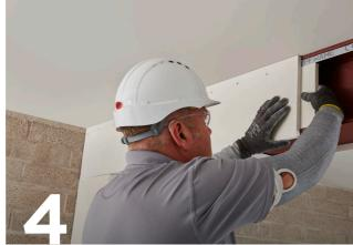
To seal the joints of single layer steel beam encasements, install additional strips of Glasroc F FireCase behind the ends of the fascia board.
