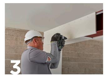
Where Glasroc F FireCase boards abut fix together with Glasroc F FireCase Screws. For four-sided protection to steel columns, Glasroc F FireCase boards are positioned and fixed board to board using Glasroc F FireCase Screws.
