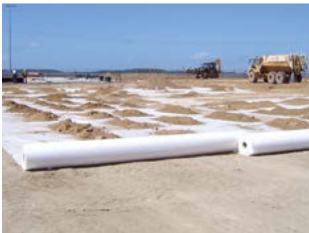
Fig. 3 Combigrid® installed as base course reinforcement where multi-directional stiffness is of great importance
