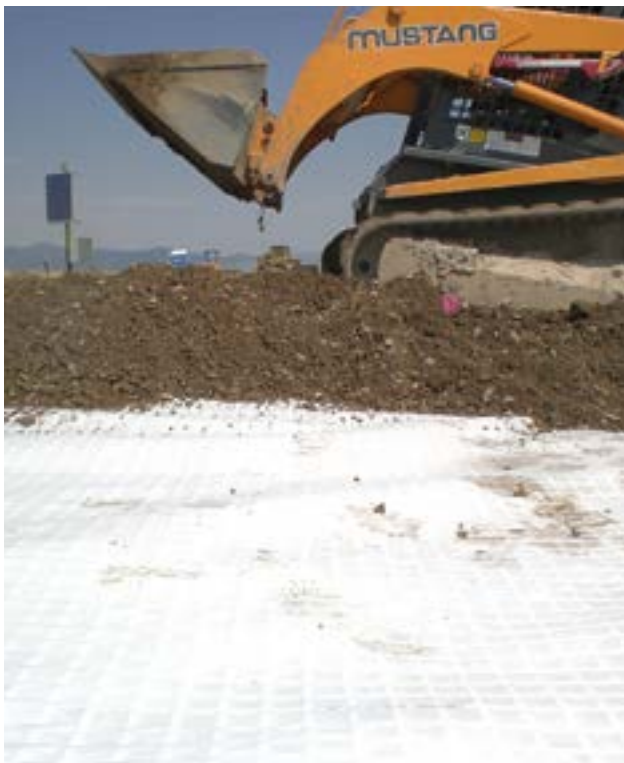
Fig. 11 Base course aggregate installed over Combigridd® for improved roadway performance
