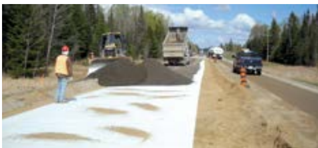
Fig. 9 Combigridd ® used over a soft subgrade to achieve soil reinforcement and soil separation and filtration to ensure long-term performance
