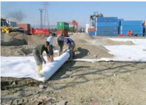
Fig. 13 Unrolling and overlapping of Combigrid® over a soft subgrade
