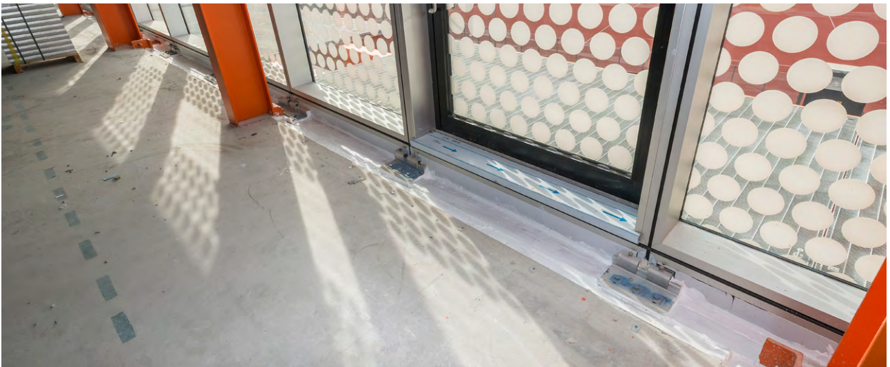
SoftSeal installed as a linear joint seal
