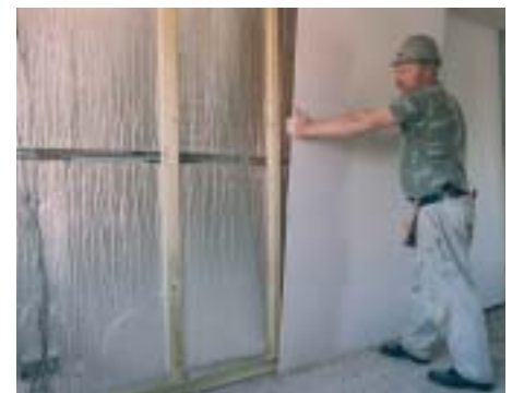
Alreflex 2L2 FR as dry lining insulation and vapour barrier
