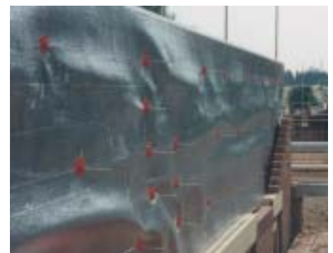
Alreflex 2L2 FR as cavity insulation/rain barrier
