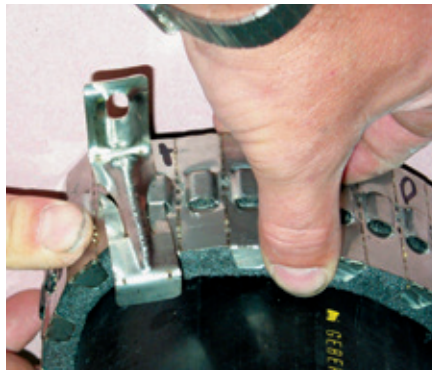
Step 5 - Fit collar around pipe
