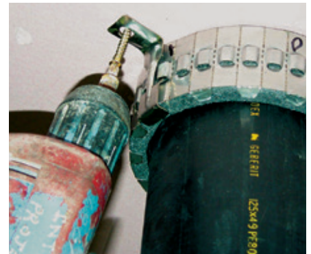
Step 6 - Secure collar in place
